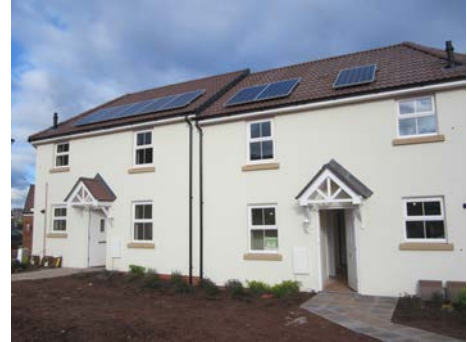
Picture 12 Photo-voltaic roof panels
