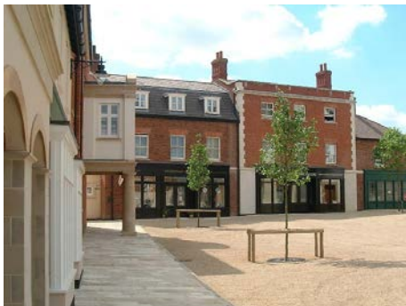
Picture 37 Commercial uses at ground floor with residential above
