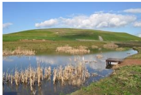
Picture 22 Example of a balancing pond
