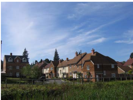
Picture 31 Dwellings side onto the open space
